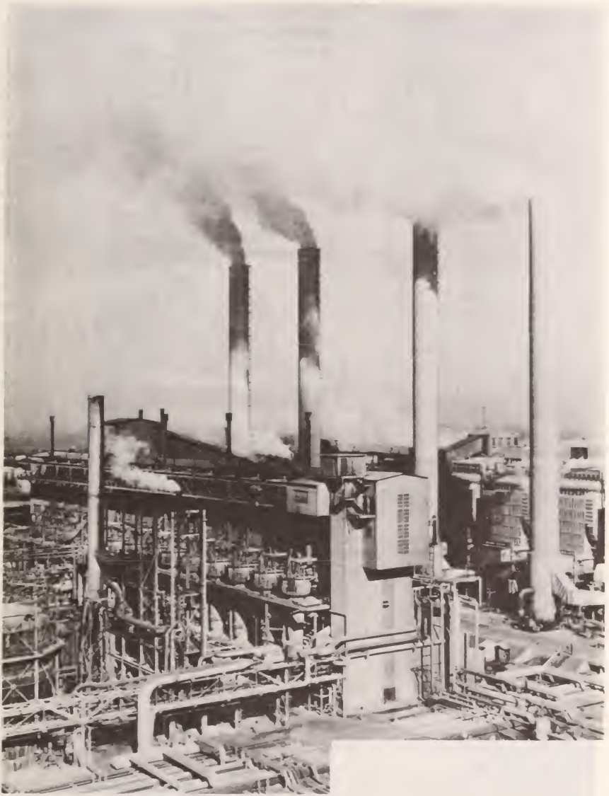
FIGURE 2.—Lurgi coal gasification building—Steam generation in background.
